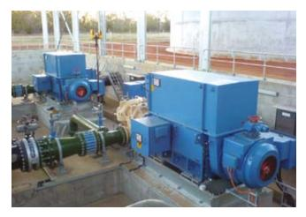
Supply: 2000 kW, 11,000 V, 4 poles, frame 560 Application: Water pumps
